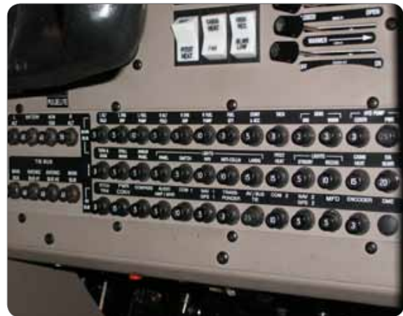
[그림 2-80] Light aircraft circuit breaker panel
