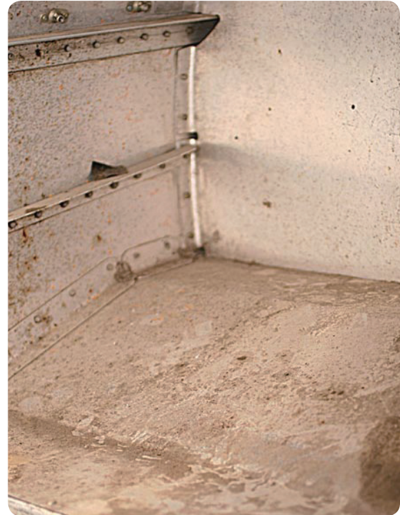
[그림 6-2] Direct chemical attack in a battery compartment
